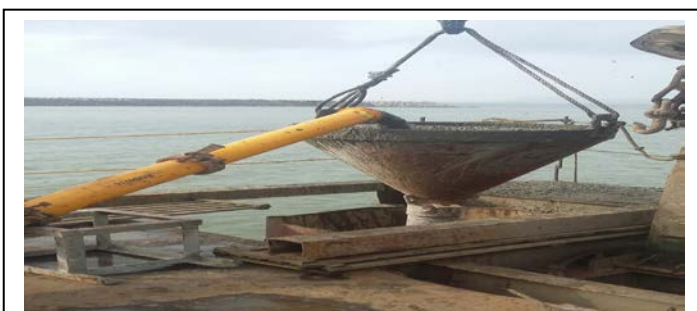
Fig. 19. Bailer, one way opening 0.5m3 capacity
