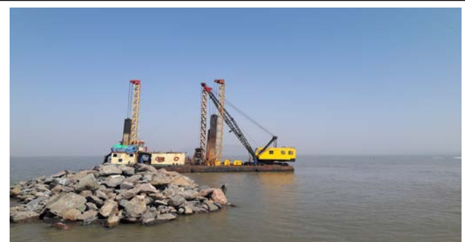
Fig. 5. First projection of breakwater above MSL
