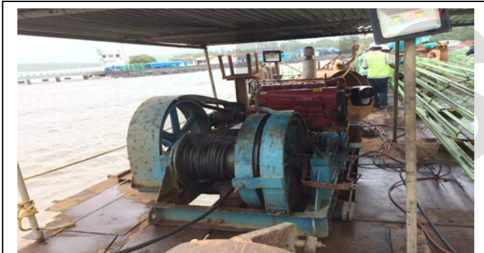
Fig. 18. Winch arrangement on the gantry crane
