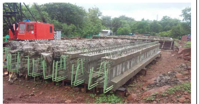
Fig. 21. Pre-caste of structure units
