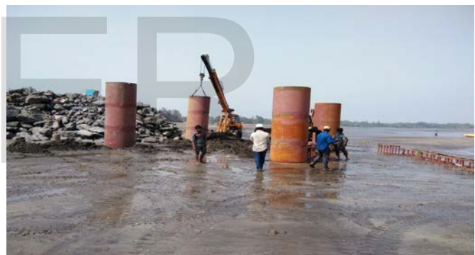
Fig. 14. Arrangement of actual and temporary pile liners
