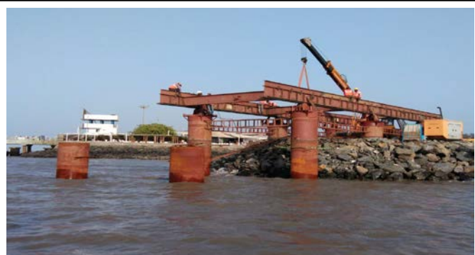
Fig. 15. Constructing and placing the gantry crane on the pile liners
